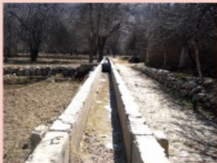
Figure 3.2 Water conservation through Water Storage Reservoir/Channel Lining
